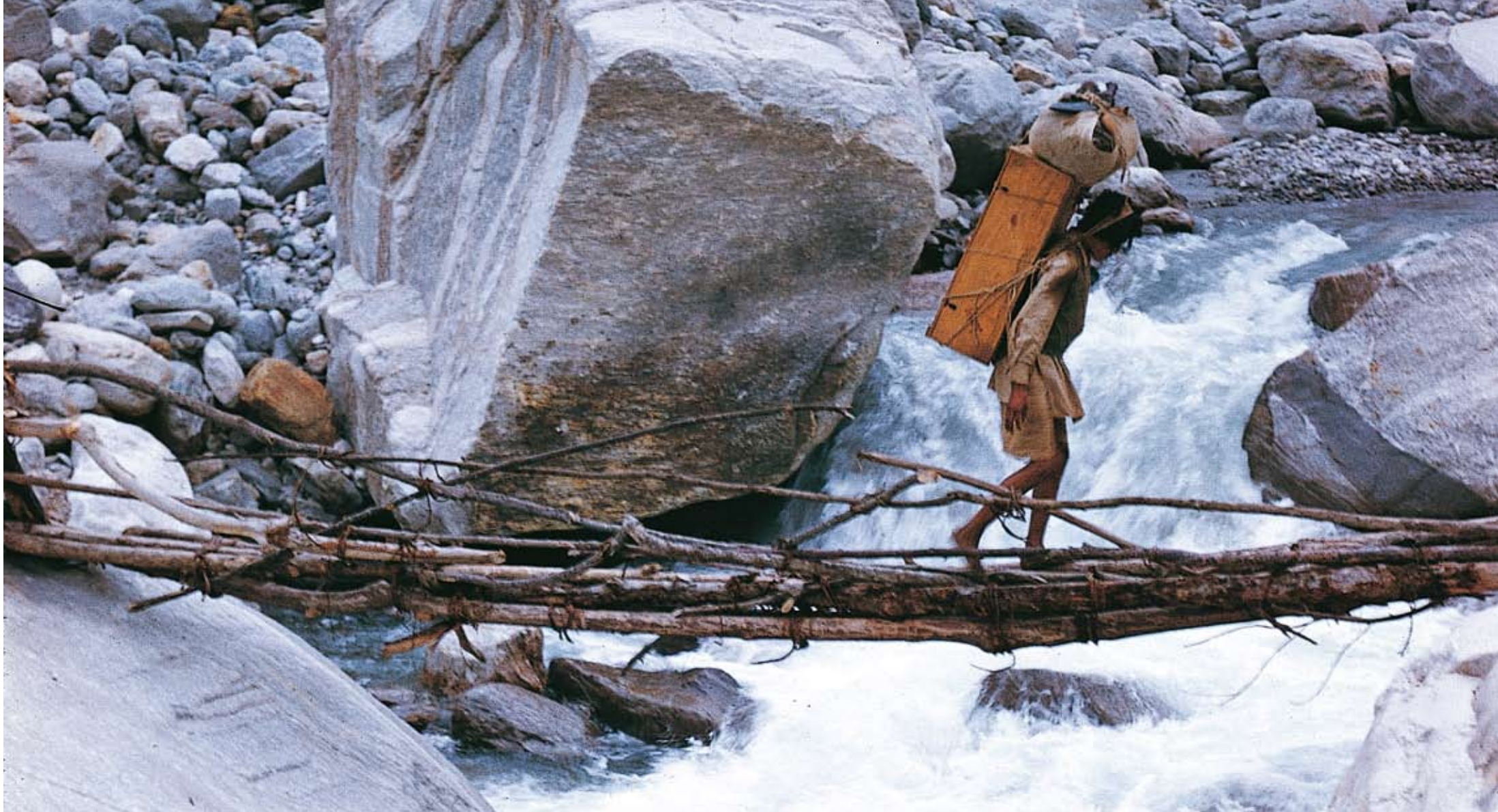
Porter crossing a makeshift bridge of tree poles tied together and resting on rocks on either side. Floods often sweep away such bridges during the monsoon, but can be easily replaced.
