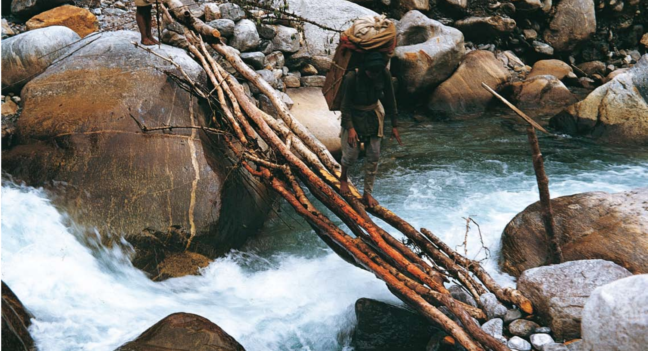
A porter balances himself while crossing a phatke (literally 'jump-over') bridge over a swift hill stream. The poles rest on the rocks on either end.
