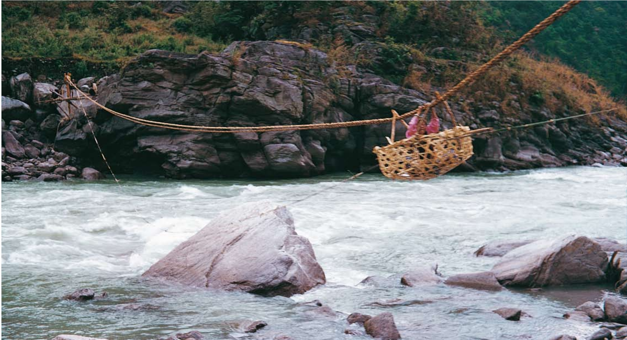
A hill woman crossing the river in a tuhin (indigenous ropeway) made entirely of local material. The thick rope is probably made from the fibre of babiyo ( Eulaliopsis binata ) or hemp ( Cannabis sativa ), and the basket is made of bamboo. The small ropes tied to the basket on either side are pulled to induce movement.
