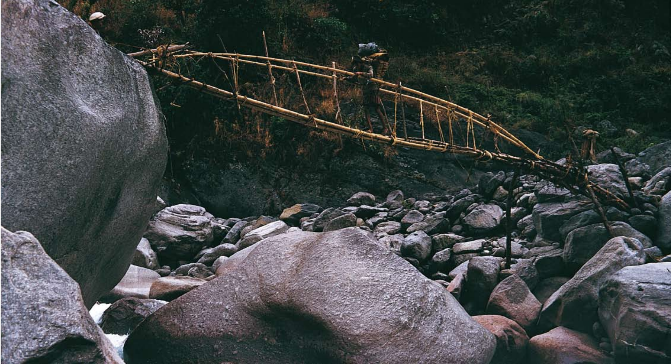
A suspension bridge with hand rails made entirely of bamboo. The span is supported by a wooden pillar on the right. The bridge rests on rocks at both ends.
