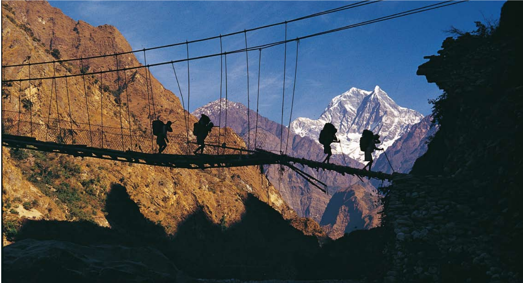
Silhouette of porters crossing the suspension bridge over the Kali Gandaki River at Tatopani along the historic Kali Gandaki trail. Suspension bridges such as this made life easier for porters along all the major hill trails. The problem of maintenance (right) was often solved using local resources and a little ingenuity. The peak in the background is Nilgiri (7061 m).
