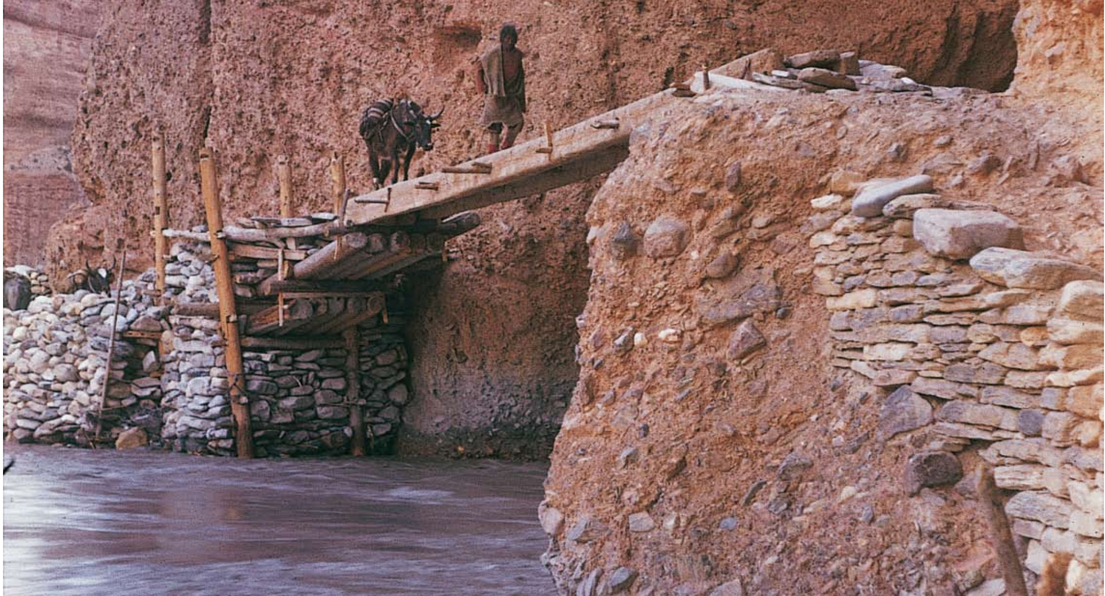
A man and his goods-carrying jhopa (cross between yaks and cows) on a wooden bridge in the trans-Himalaya region. The cantilevered timber stacked one atop the other at both ends support the span in the middle.
