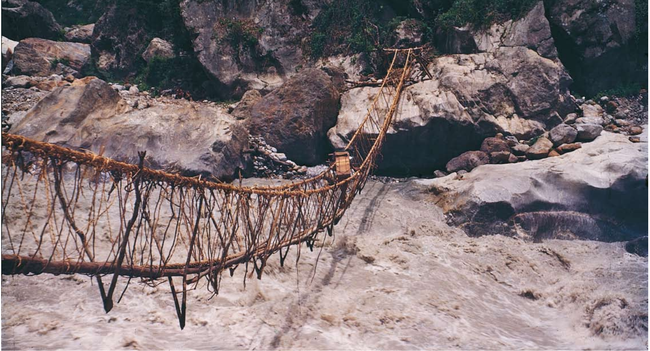
A porter crossing a raging Himalayan torrent on an indigenously built suspension bridge in the eastern mountains. The bridge is anchored to poles fixed on large rocks on either side. V-shaped tree branches, ropes and vines hold the poles that are used for stepping at the base.
