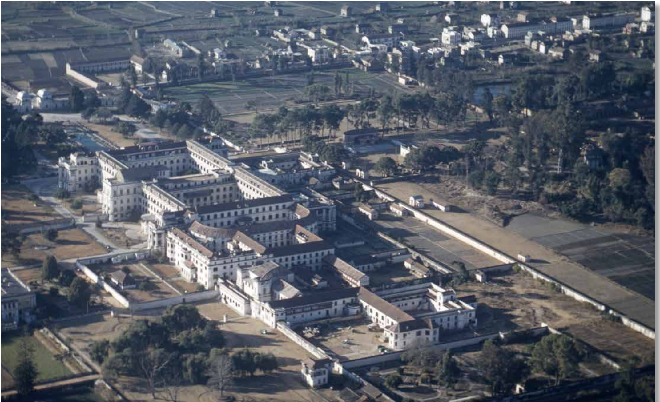
Aerial view of Singha Durbar, the then resident palace built for Rana prime-minister amidst fertile fields of Kathmandu during the year 1903 AD converted into central government secretariat after 1950. Currently it is covered by the concrete jungle of urban Kathmandu leaving no fields for agricultural practices.
