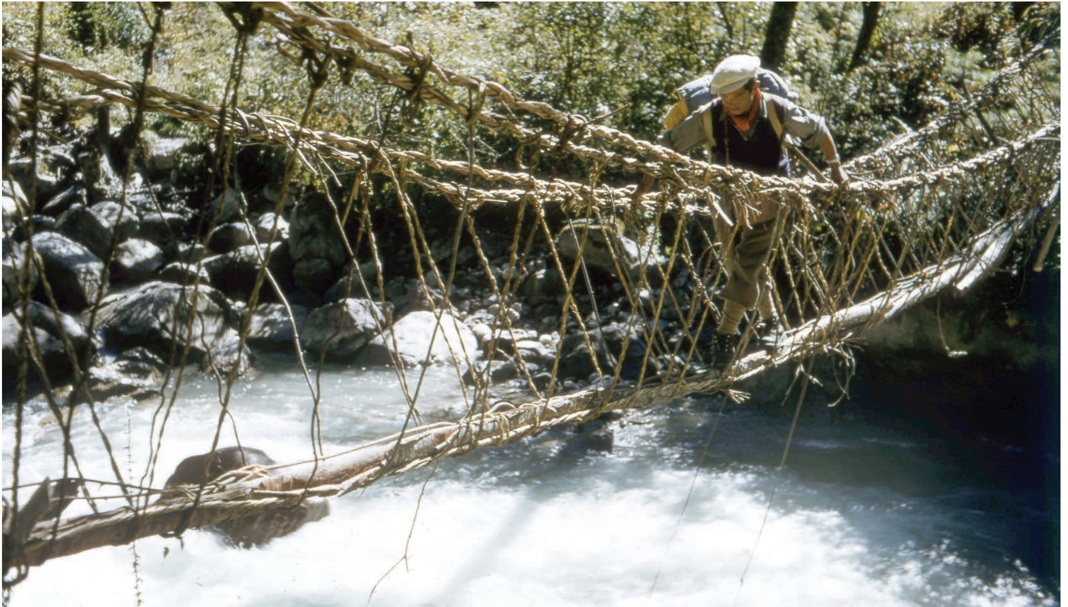
Suspension bridge made of choya (bamboo splints) in a side valley of near the Arun River. Such bridges were fragile and prone to breakage. Despite the risks, people used the bridge in their daily life as there was no other way to cross rivers.
