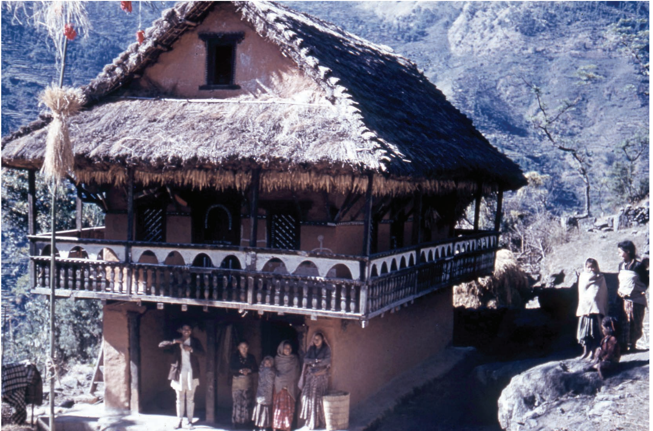
A traditional Limbu house near Taplejung. The house is made of stones using mud mortar, with locally available wood and roofing thatch, has corncobs hanging to dry under the eaves.
