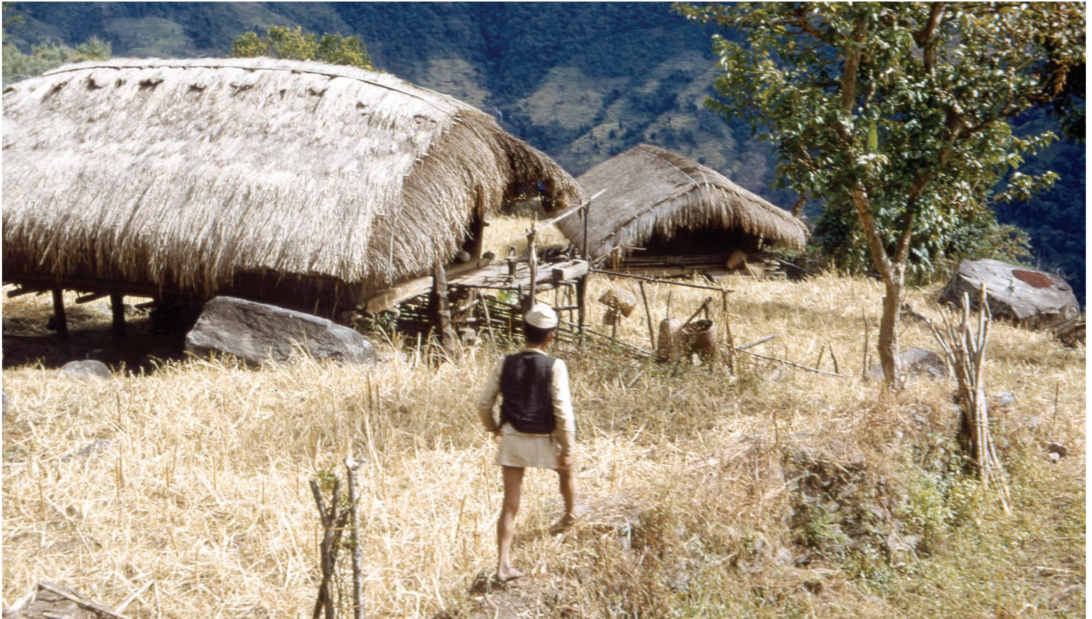
A peasant in a Rai village walks towards his barn built on wooden piles, raised about five feet from the ground and accessible via a wooden ladder through a front verandah. The walls were made of bamboo and topped with a thatched roof. The barns were occasionally used for shelter by people also.
